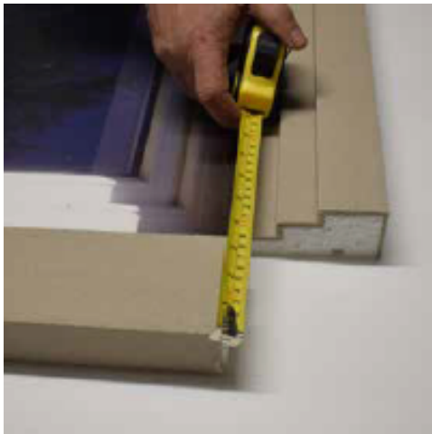
5. Measure side reveal width
