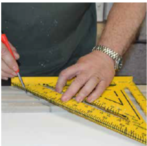
7. Mark mitred edge on side reveal
